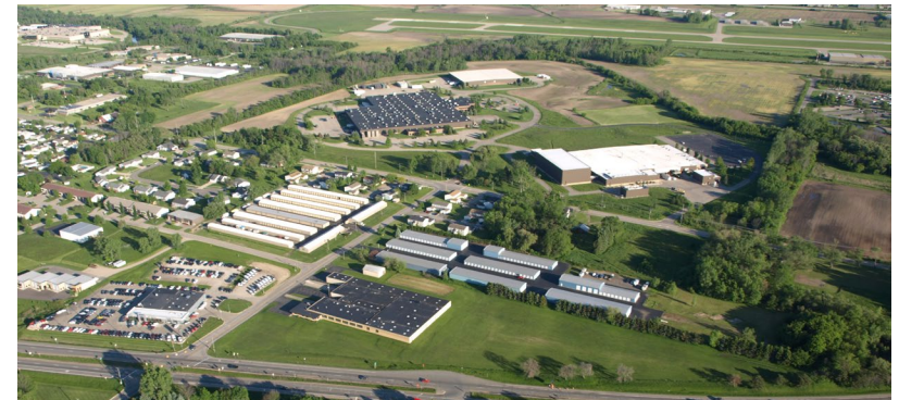
The Industrial areas on the Future Land Use Map provide for the preservation and development of larger-scale industrial uses.
